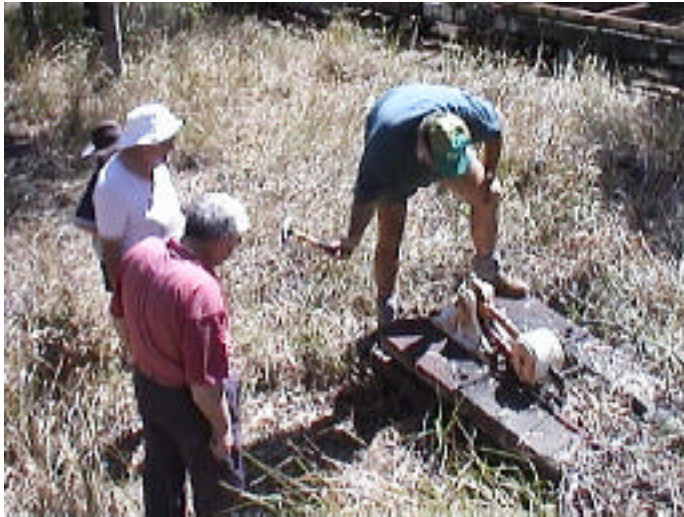
Left: Removing the Point Lever from the sleeper near Herb Garden end.
