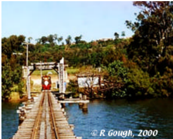
Above – Lift Span River Bridge, Maroochy River, 2000 – Photo R Gough
