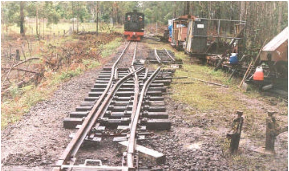
Points in position at the start of a wet day's work. The curve in the points was removed by jacking and barring across during the day. The panel of
