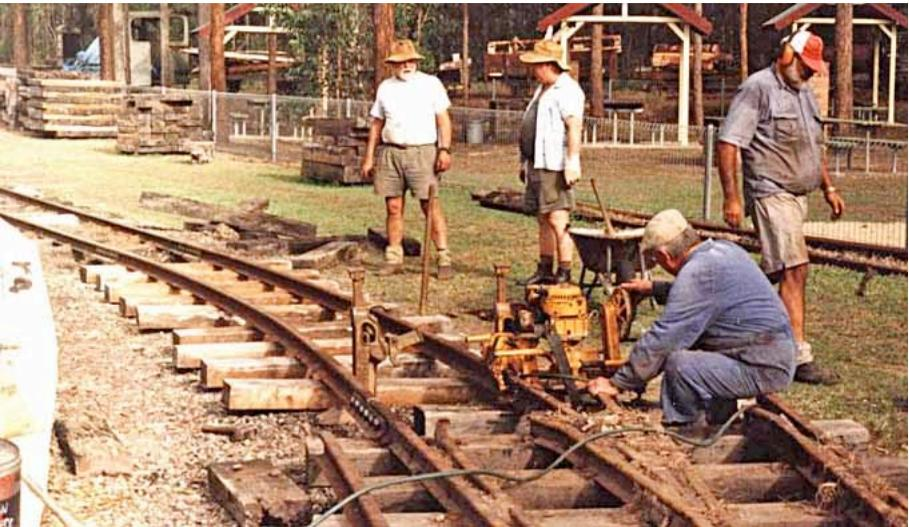
Points at Margaret Street end of passing loop - Leslie Beahan using motorised rail drill to drill fishplate holes to allow points to be connected to existing mainline. Bill Blannin photo [bb280\_1]
