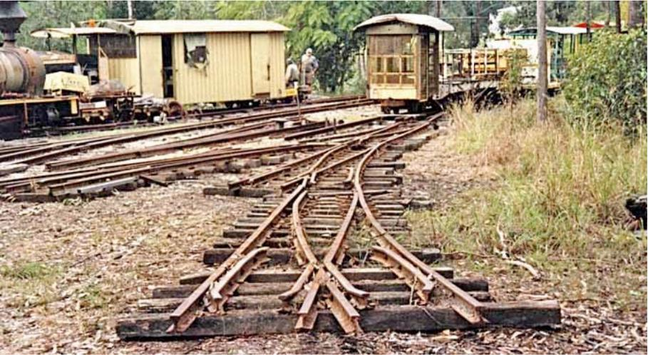
Pointwork roughly placed for the southern end of the passing loop and access to the compound. Bill Blannin photo [bb280\_2]
