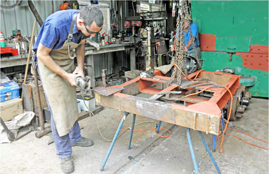
Mark Gough grinding and welding the bogie from the Nambour wagon, January 2011. Bob Gough photo.
