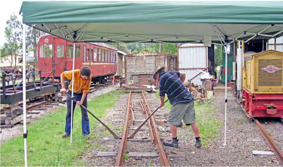
Dave and Ryan dismantling the workshop area's storage siding in preparation for the new service track, 12 December 2010. Terry Olsson photo.
