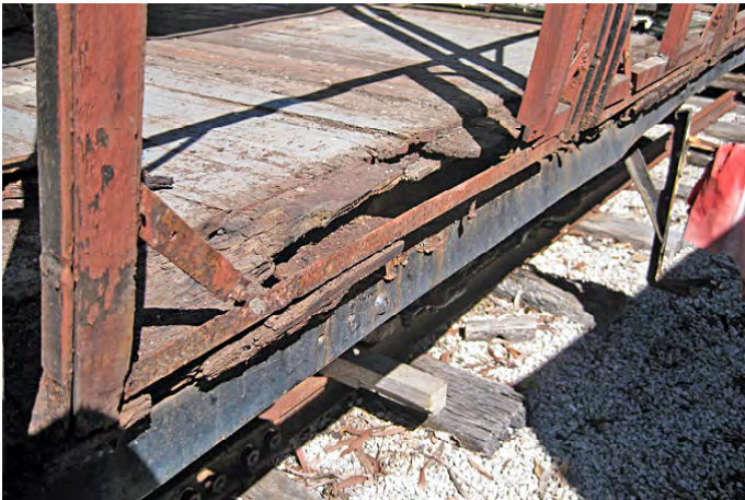
The badly deteriorated timbers along the side of the RM trailer show why PL111 was withdrawn from service for its current repairs. Terry Olsson photo.
