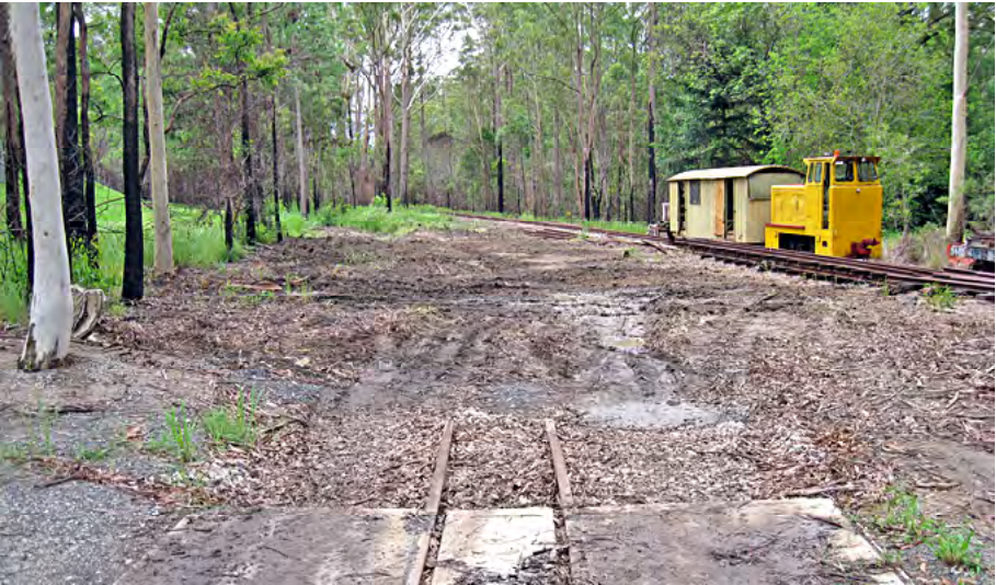
Site of the new Storeybrook Station, cleared 16 February 2013. Terry Olsson photographer.
