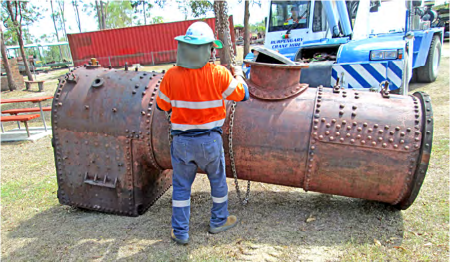
Removing Bundy's boiler for scheduled maintenance, 11 January 2013. Ryan Silk photographer.
