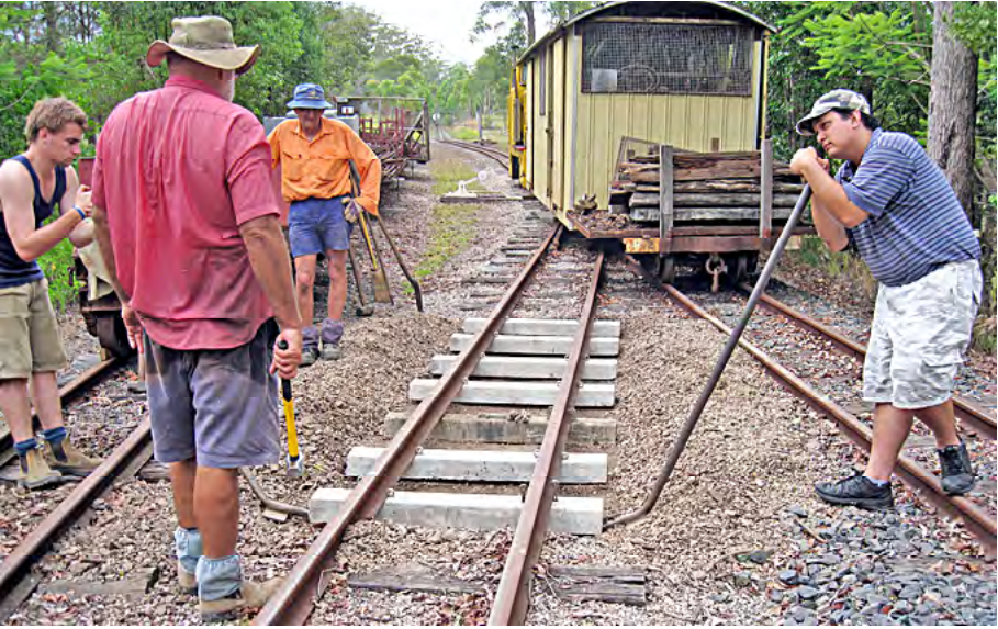
Installing Mackay concrete sleepers in crossover to Workshop, 5 January 2013. Terry Olsson photographer.
