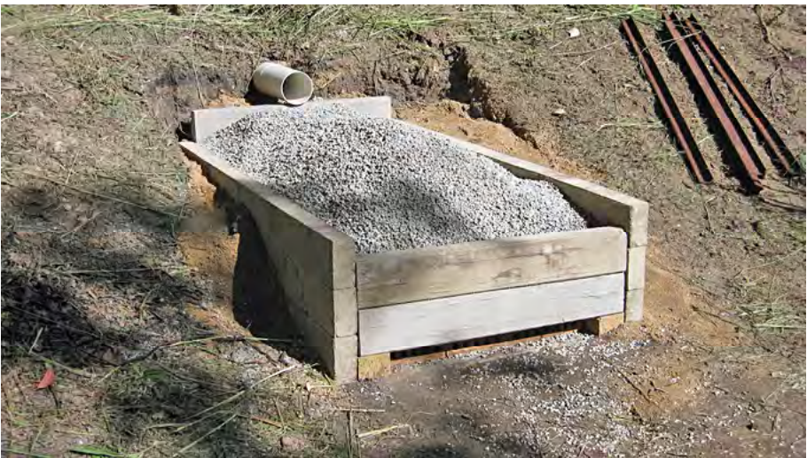
Greg Stephenson assembling the filter drain on the stormwater outlet from the elevated inspection track, 13 May 2013. Terry Olsson photographer.
