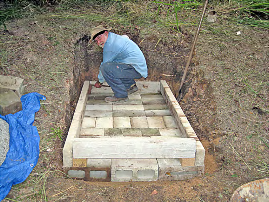
Greg Stephenson assembling the filter drain on the stormwater outlet from the elevated inspection track, 13 May 2013. Terry Olsson photographer.
