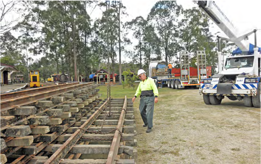
Unloading some of the fifteen panels of rail on concrete sleepers transported from Ingham, 26 August 2013. Ryan Thomas photographer.
