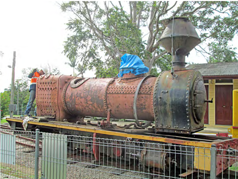
Lift off!. Melbourne's boiler being removed as restoration continues. May 2014 Ryan Thomas photographer.
