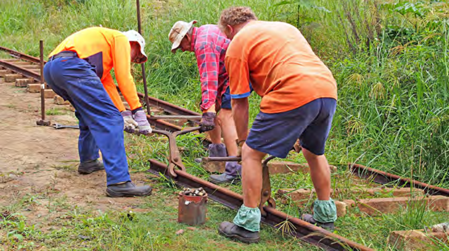
Kerry Rasmussen, Steve Baker and Dave Carusso positioning a rail before lifting it onto the sleepers, 14 June 2014. Sue Rasmussen photographer.
