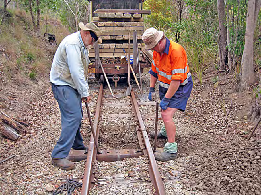
Greg Stephenson and Dave Carusso (above) using hooked lifting bars to move and place the 100th steel or concrete sleeper on the existing main line and the sleeper in place (below). Terry Olsson photographer.
