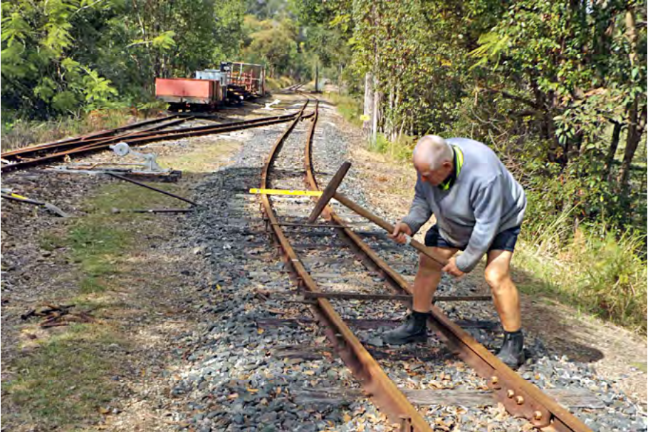
Re-spiking timber sleepers for mainline maintenance: Dave Pearson with spiking hammer, 27 June 2015. Greg Stephenson photographer.
