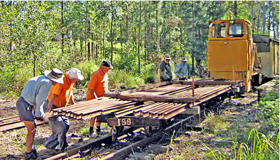
Manually shifting lengths of rail during a trackwork party, August 2008. Bill Blannin photographer.
