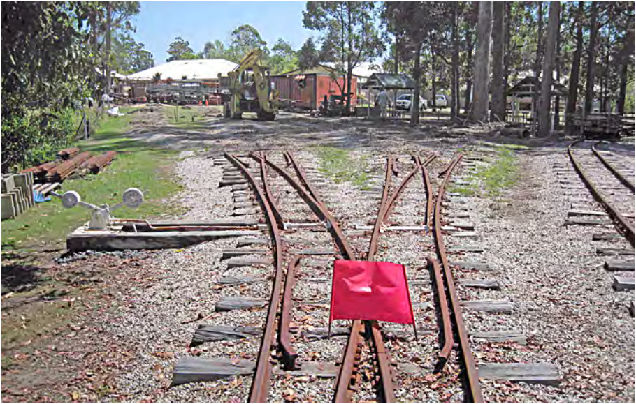
Storage sidings removed and points closed by "red board". These points will be raised to future levels to access the storage shed by increasing the depth of ballast. Terry Olsson photographer.
