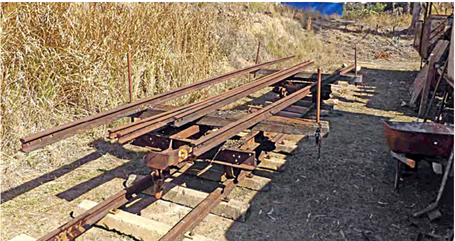
Bolster wagon of rails ready to be placed onto the concrete sleepers. Greg Stephenson photographer.
