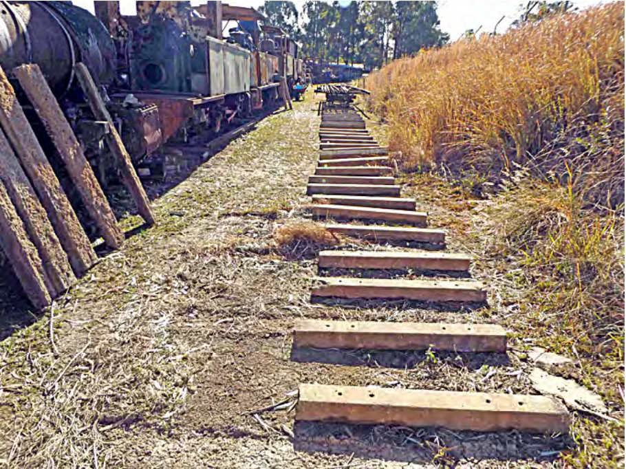
Concrete sleepers in place with bolster wagon of rails ready to be placed onto the sleepers. Greg Stephenson photographer.
