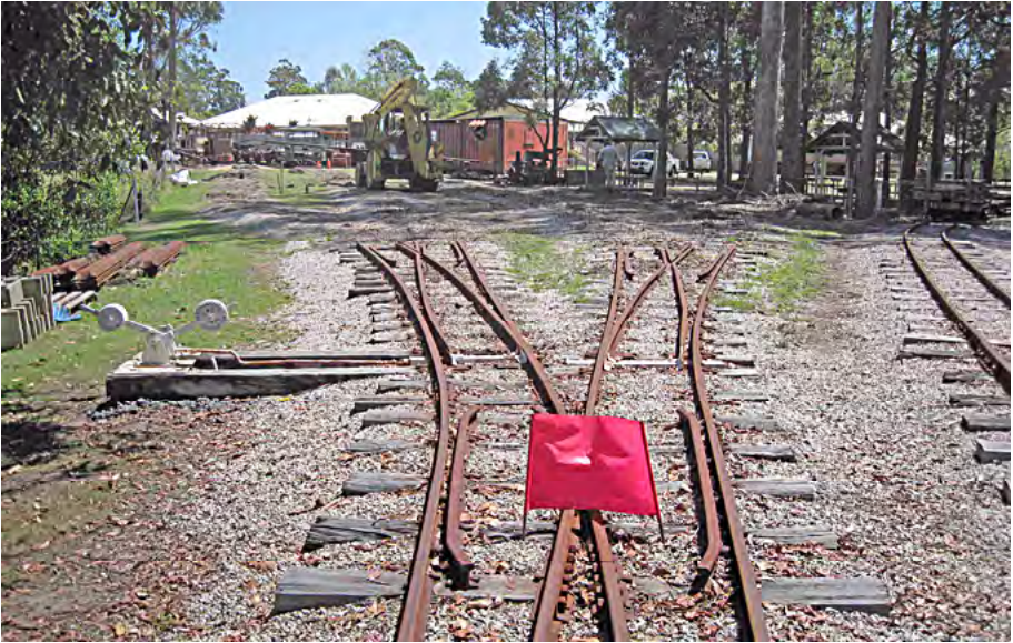
Storage sidings removed and points closed by "red board". These points will be raised to future levels to access the storage shed by increasing the depth of ballast. Terry Olsson photographer.
