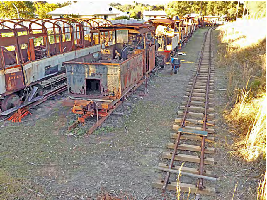
Another view of the completed storage siding ready for placing of rolling stock from the area of the new shed. Greg Stephenson photographer.
