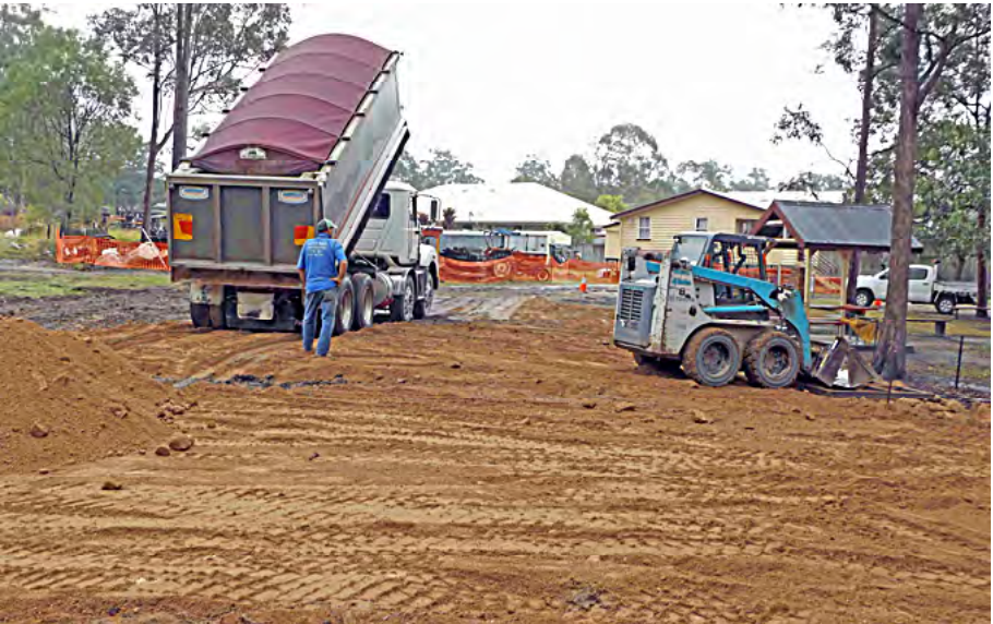
Above: Another load of decomposed granite (“deco”) fill arrives as the bobcat is used to remove the grass from the area to be filled. Thursday, 16th June, 2016. Below: A levelling frame was used on the bobcat to spread and shape the fill. Thursday, 16th June, 2016. Greg Stephenson photographer.
