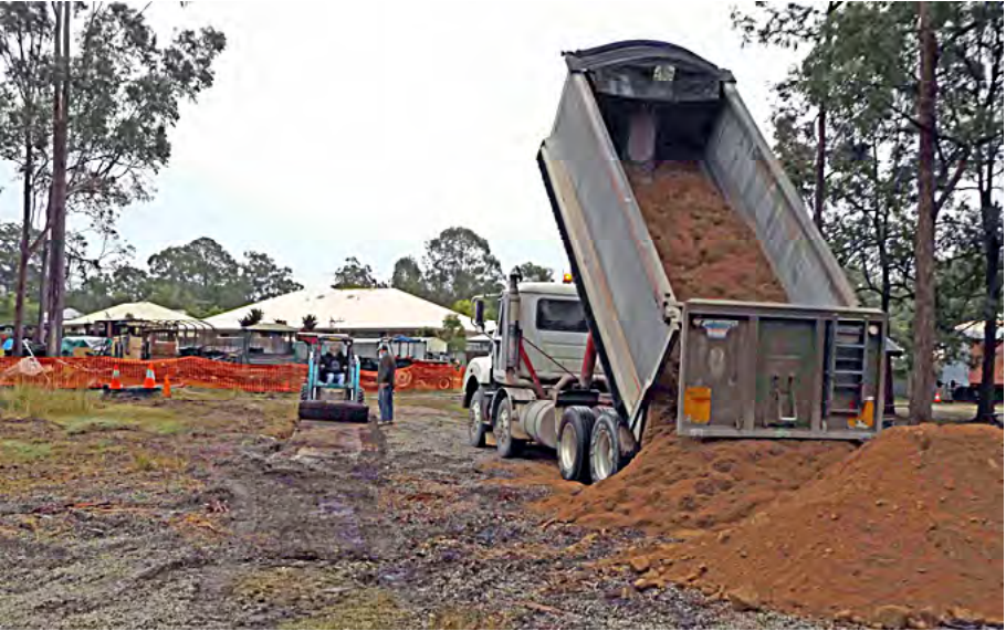
Above: Another load of decomposed granite (“deco”) fill arrives as the bobcat is used to remove the grass from the area to be filled. Thursday, 16th June, 2016. Below: A levelling frame was used on the bobcat to spread and shape the fill. Thursday, 16th June, 2016. Greg Stephenson photographer.
