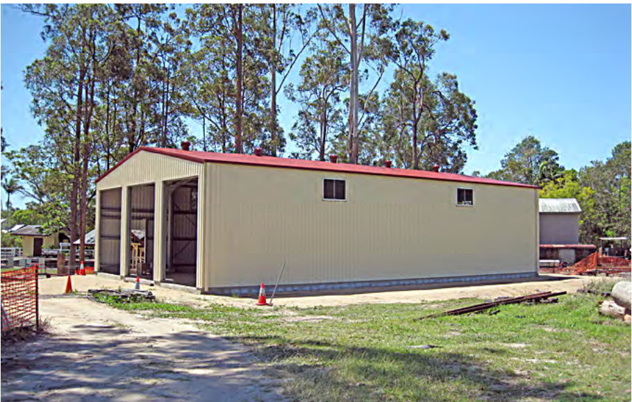
Loco shed construction, 2 October 2016. Terry Olsson photographer.
