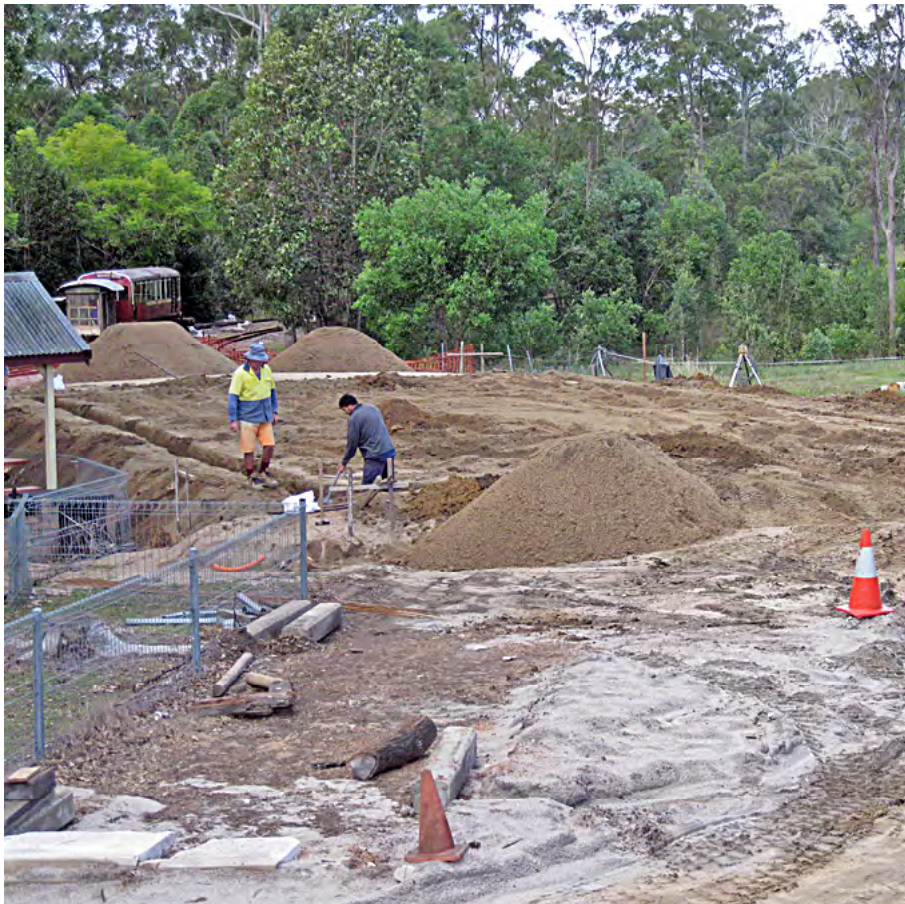
ANGRMS' shed site preparation, 22 June 2016. Terry Olsson photographer.
