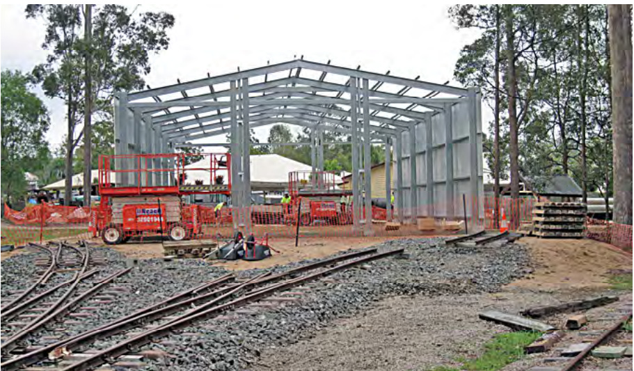
ANGRMS' loco shed construction, 15 September 2016. Terry Olsson photographer.
