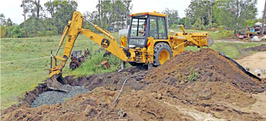
Above: Ralph Cumner commences backfilling of one of the roof water drainage pits for the locomotive storage shed. Greg Stephenson photo. Below: New members Barry and Bill help Greg laying track within loco shed A, 28 January 2017. Terry Olsson photographer.
