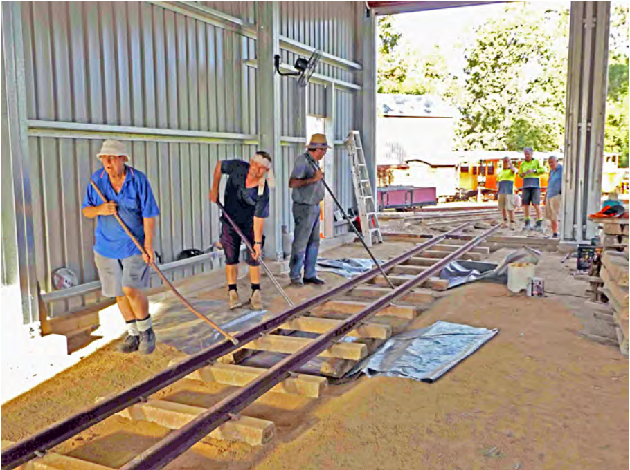
Bob Gough, Wayne Harmen and Morrie Mason using crow bars to adjust the alignment of the track panels prior to concreting the floor of the locomotive storage shed. Greg Stephenson photographer.
