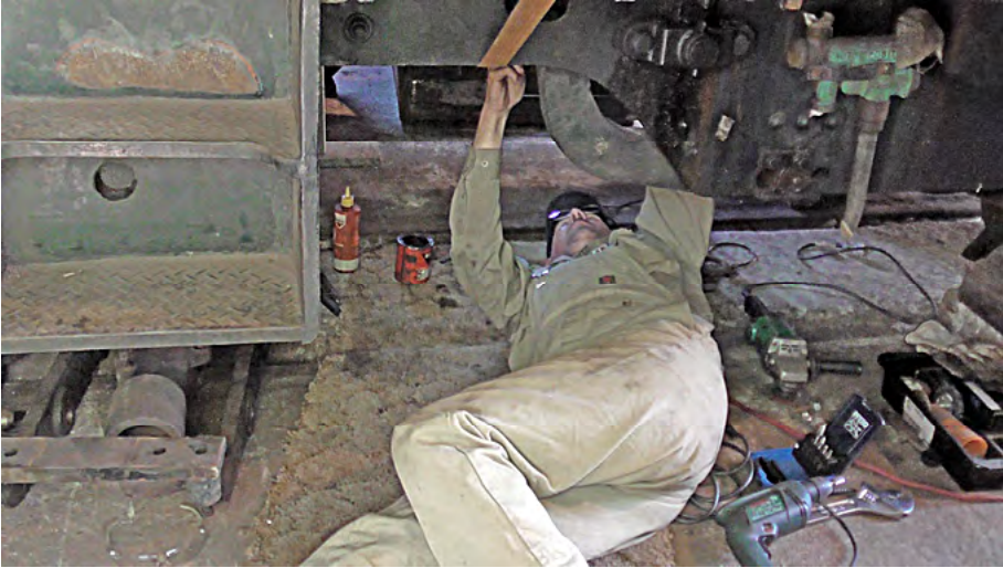
Mark Gough working on the ash pan of the Perry Loco, replacing worn out pivot pins with those made on his home lathe. Bob Gough photographer.
