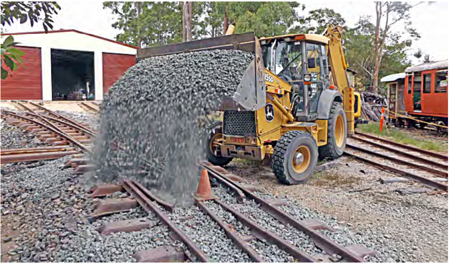
Above: Ralph Cumner helping to place ballast on the tracks approaching the locomotive storage shed. Below: As concrete pours from the pipe from the concrete pump it is vibrated around the track and sleepers. The temporary timber boards to form the flangeways for the railway wheels can be seen supported beside the rails. Greg Stephenson photographer for both photos.
