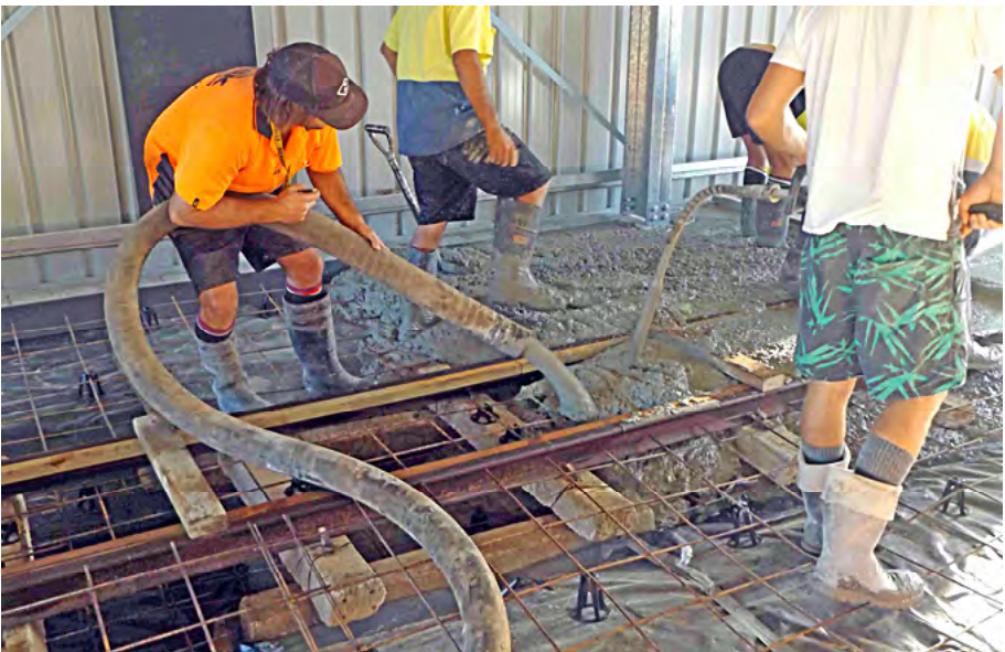
Above: Ralph Cumner helping to place ballast on the tracks approaching the locomotive storage shed. Below: As concrete pours from the pipe from the concrete pump it is vibrated around the track and sleepers. The temporary timber boards to form the flangeways for the railway wheels can be seen supported beside the rails. Greg Stephenson photographer for both photos.
