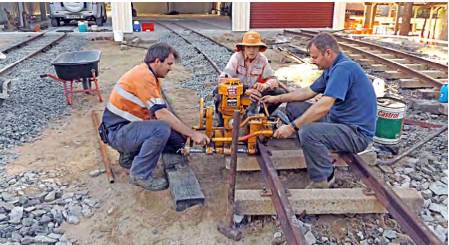
Ryan Thomas, Harrison Silk and Wayne Harman using the rail drill to make fishplated joints on Number 2 road, 3 June 2017. Greg Stephenson photographer.
