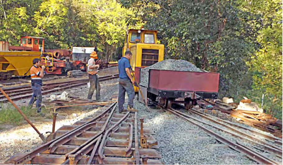
"Gemco" was used to bring a load of ballast in the ex-Douglas Shire Tramway wagon along Number 1 road so that points between Number 2 and 3 roads can be ballasted. The pointwork has been lifted to the correct height and supported on jacks, 3 June 2017. Greg Stephenson photographer.
