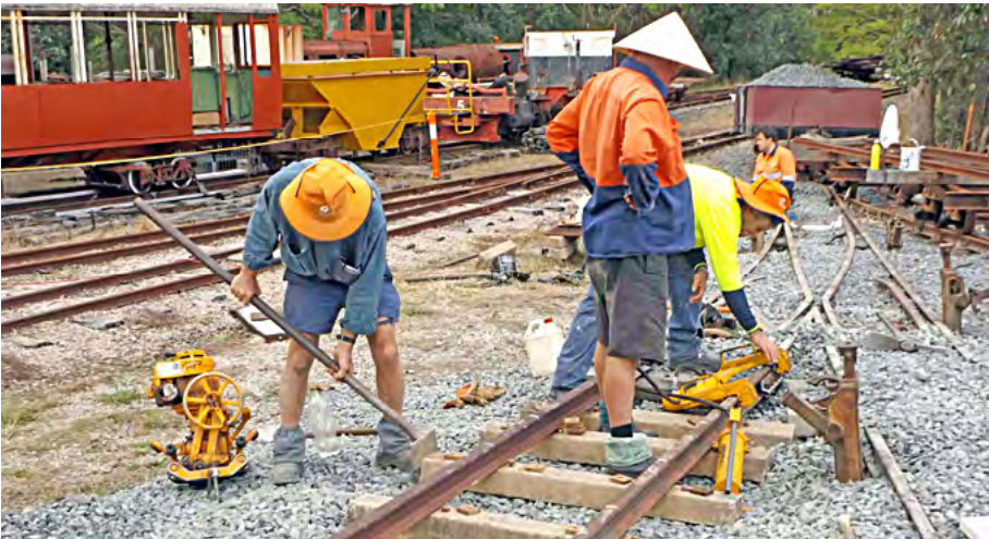
Steve Baker uses a bar to adjust the position of ex-Ingham concrete sleepers on Number 3 road, whilst Dave Caruzzo and Terry Olsson use the hydraulic rail bender to adjust the alignment of the rails at the joint, 17 June 2017. In the background, Ryan Thomas is fitting rods to the point levers. Greg Stephenson photographer.
