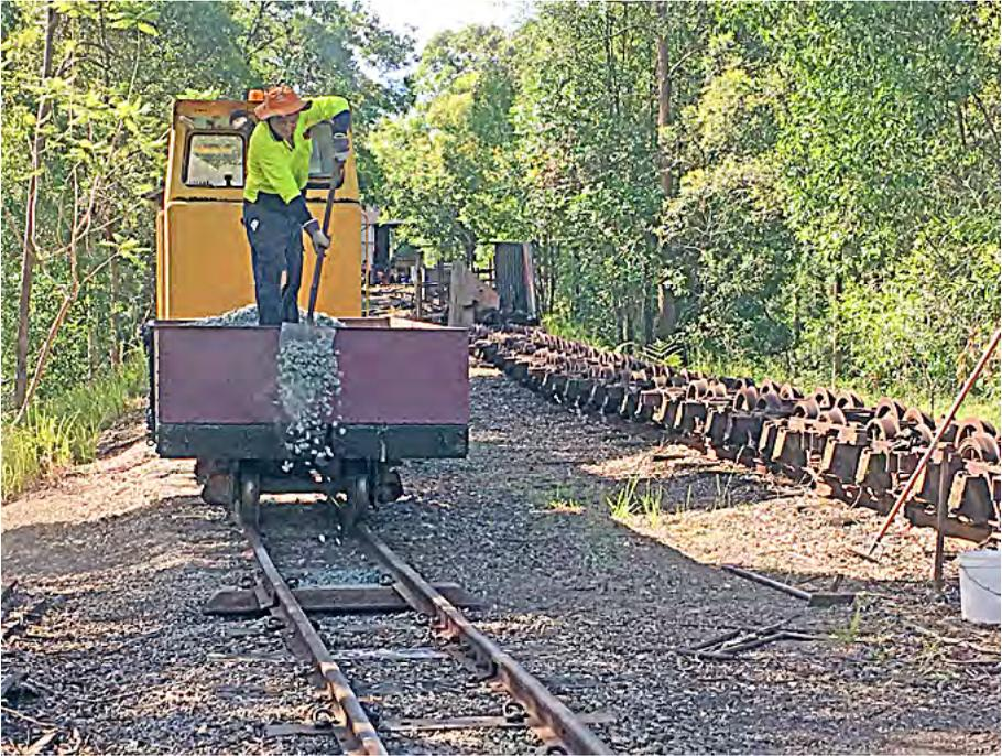
Terry Olsson unloads ballast, 23 December 2017, to pack steel sleepers installed to replace the cluster of defective timber sleepers identified during the annual independent track inspection. Greg Stephenson photographer.
