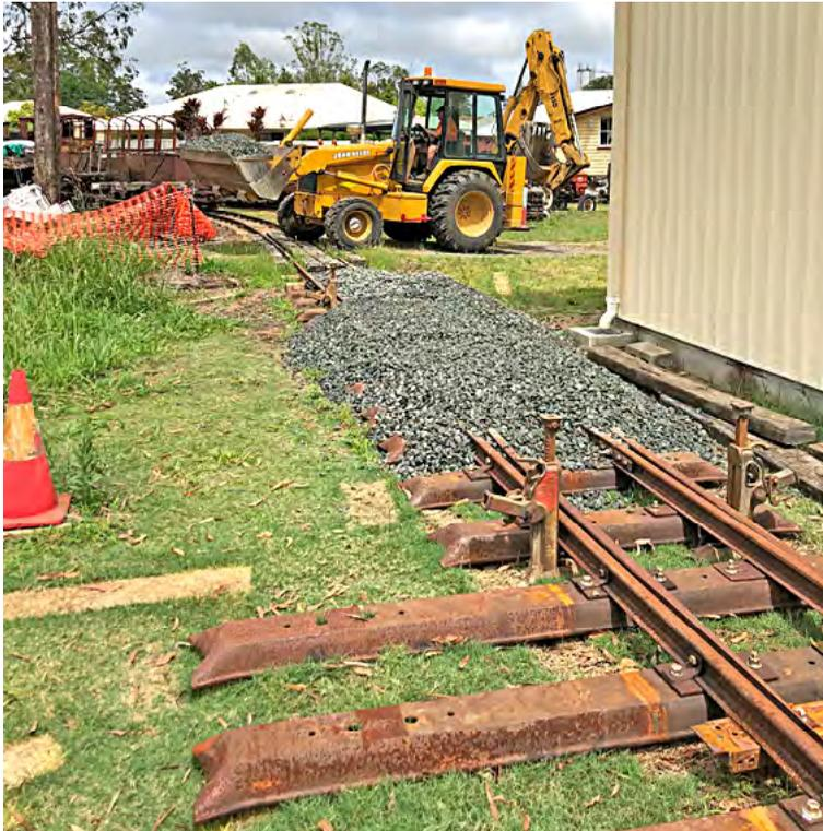
Ralph Cumner using his back hoe to carry ballast to the by-pass track beside the locomotive storage shed. The track jacks supporting the track can be seen in the foreground and the pointwork in under the ballast that has been placed. Wayne Harman photographer.
