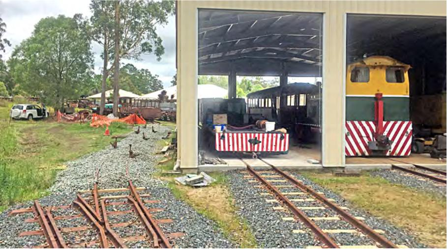
Ballast placed on the by-pass track and awaiting lifting and packing. The track jacks supporting the rails to their final levels can be seen protruding through the ballast. Greg Stephenson photographer.
