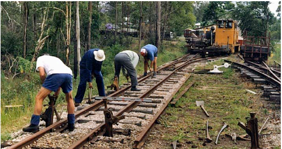
Brian Wilson, Lynn Zelmer, Bob Gough and Greg Stephenson on a typical trackwork party packing ballast under recently replaced sleepers (8 Nov 2003). Bill Blannin photo.
