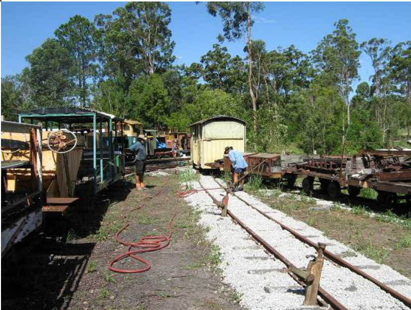
Work in progress on levelling and ballasting No.2 Road.
