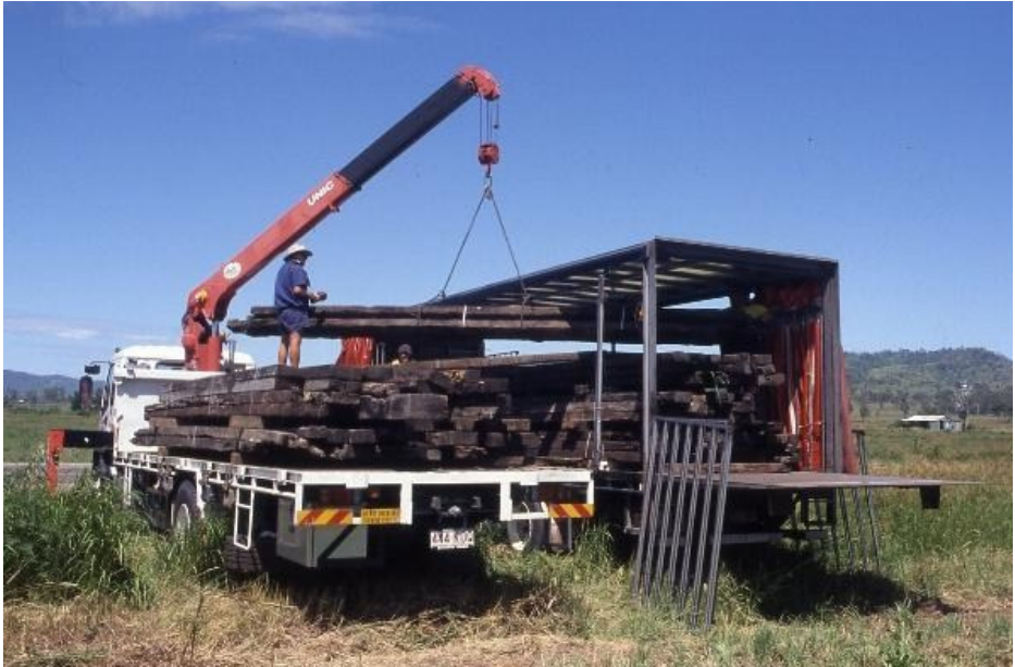
Loading bundles of bridge timber at Nindooinbah Bridge, Beaudesert.
