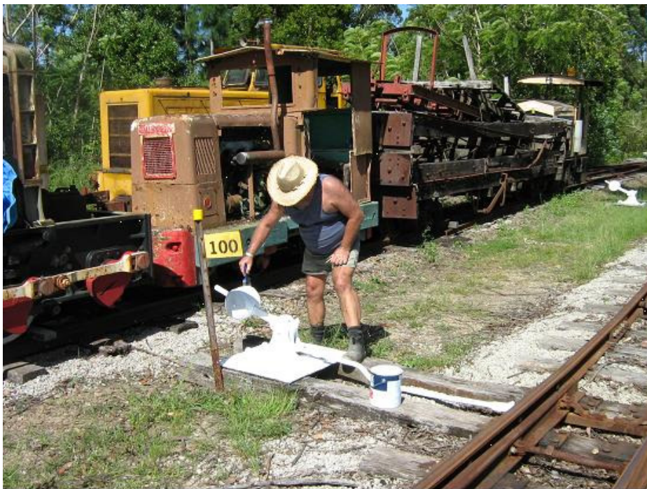
Proving that attention to detail is important, Geoff Wilson paints the point throw on the mainline points at Chainage 100. Photo: Bill Blantin
