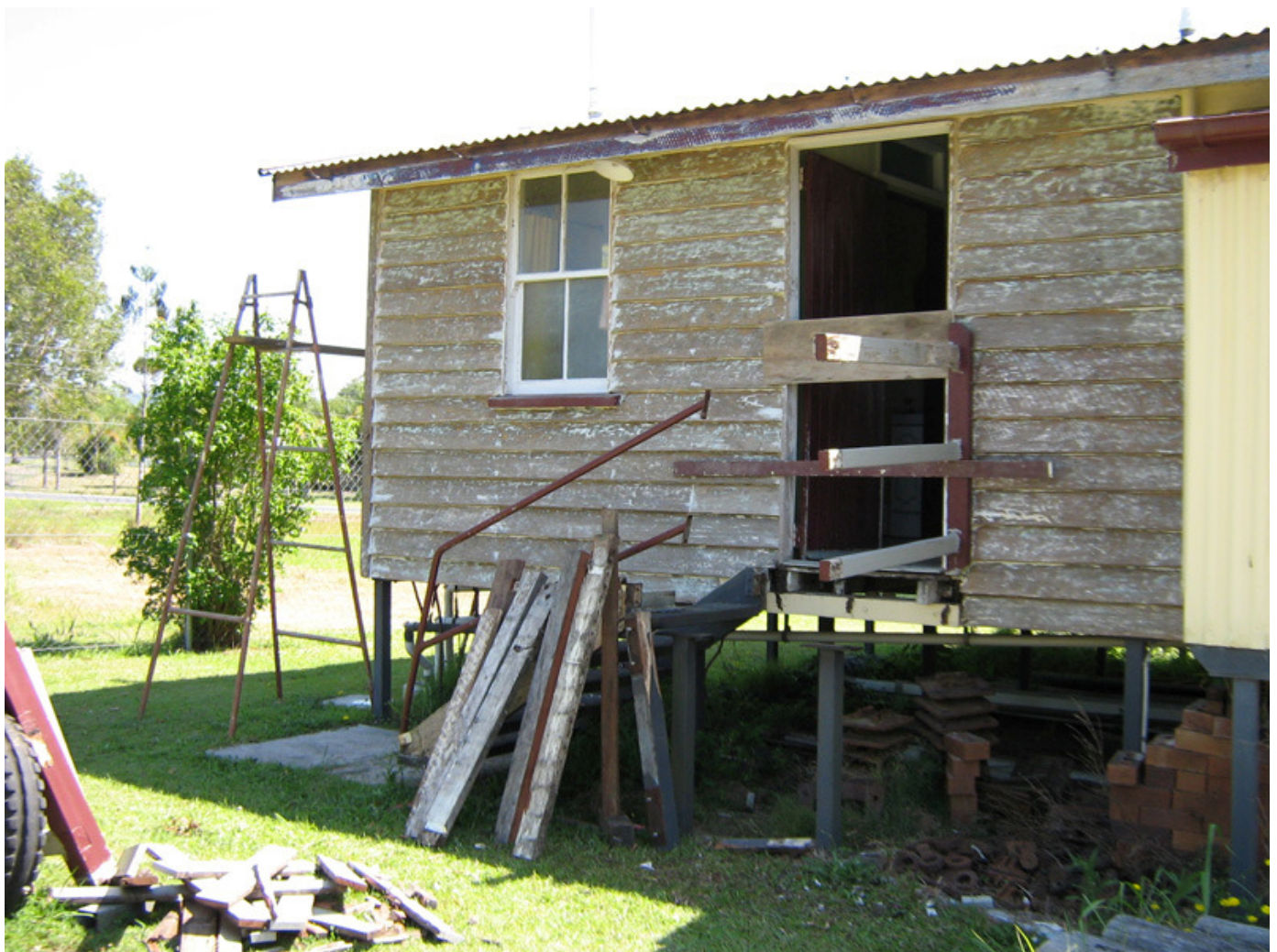
Rear of QCWA Cottage sanded back for repainting. Guttering has been removed for replacement as has the rear landing. Photo: Bill Blannin.
