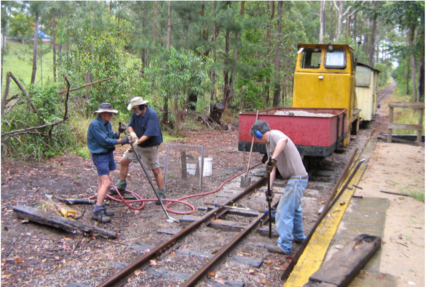
Steve Baker, Greg Stephenson and Terry Olsson replace sleepers at Storybrook Station. This section will remain as access to the rail stockpile when the new station is developed. Photo: Bill Blannin.
