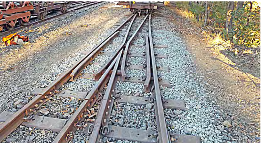
Above: Ryan Thomas replacing deteriorated bolt in the frog on the mainline points leading to the Locomotive Storage Shed. Below: Completed repairs on the mainline points leading to the Locomotive Storage Shed showing 6 steel sleepers with welded lugs and Pandrol "e" clips. Greg Stephenson photographer.
