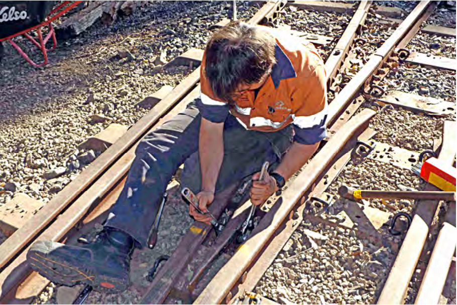
Above: Ryan Thomas replacing deteriorated bolt in the frog on the mainline points leading to the Locomotive Storage Shed. Below: Completed repairs on the mainline points leading to the Locomotive Storage Shed showing 6 steel sleepers with welded lugs and Pandrol "e" clips. Greg Stephenson photographer.
