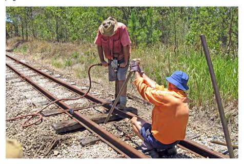
Timber sleeper being held in place against the rails by a lifting bar whilst spike holes are drilled with the air drill. The rails are held in correct position with a track gauge and sash clamp. [Iz 680]
