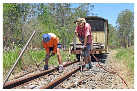
Steve Baker using a pick to push ballast under the sleeper while Greg Stephenson uses air hammer to tightly pack the ballast. To left of Steve is a screen used to remove fine material from contaminated ballast before reusing it in the track. [Iz\_735]
