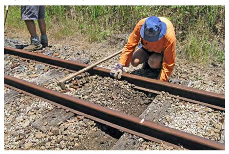
Dog spikes have been extracted and ballast removed from beside the sleeper to be replaced. The sleeper will then be knocked sideways into the cleared area so it can removed. The white chalk mark on top of the rail shows the centre location of the sleeper. [Iz\_601]
