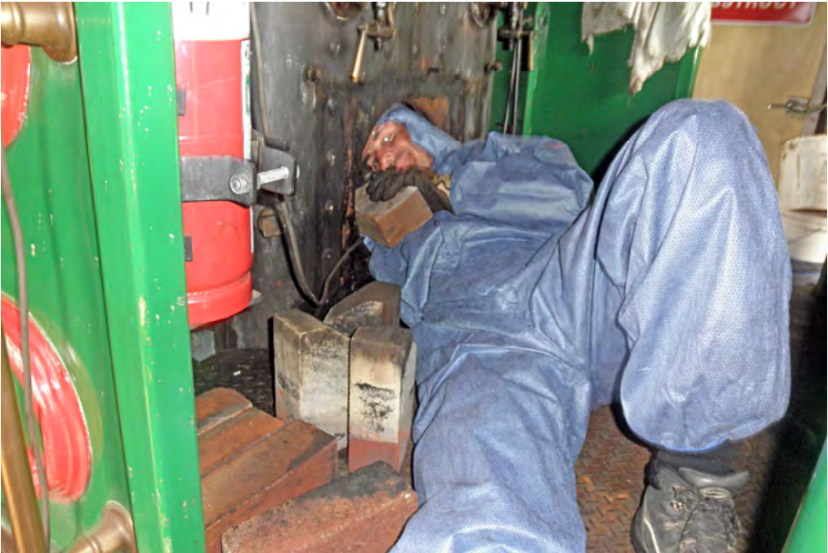
Mark Gough, removing fire box bricks from the Perry as the ex-Dreamworld loco gets a work over, 10 Jan 2015. Bob Gough Photographer.
