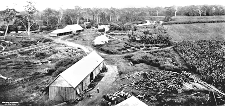
Morayfield Sugar Plantation outbuildings and sugar cane planting (right) near Caboolture, 1873 (apparently taken from top of sugar mill building). Unidentified photographer, from John Oxley Library, State Library of Queensland, negative 65889; image has been digitally enhanced.
