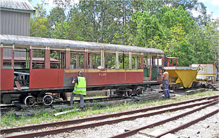
Conner and Ryan Work on RM Trailer, 16 October 2016. Terry Olsson photographer.
