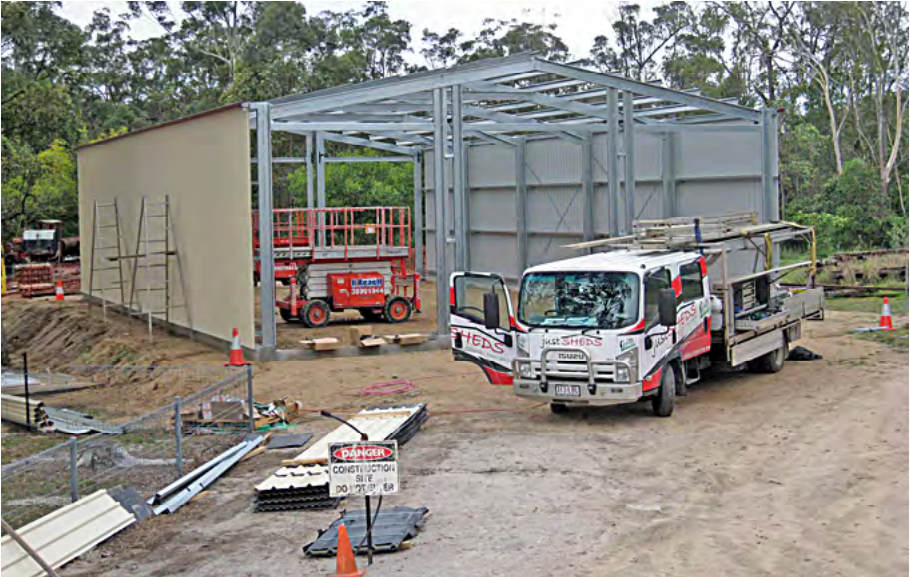
Loco shed construction, 15 September 2016. Terry Olsson photographer.
