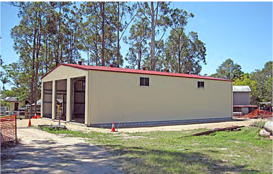
Loco shed construction, 2 October 2016. Terry Olsson photographer.
