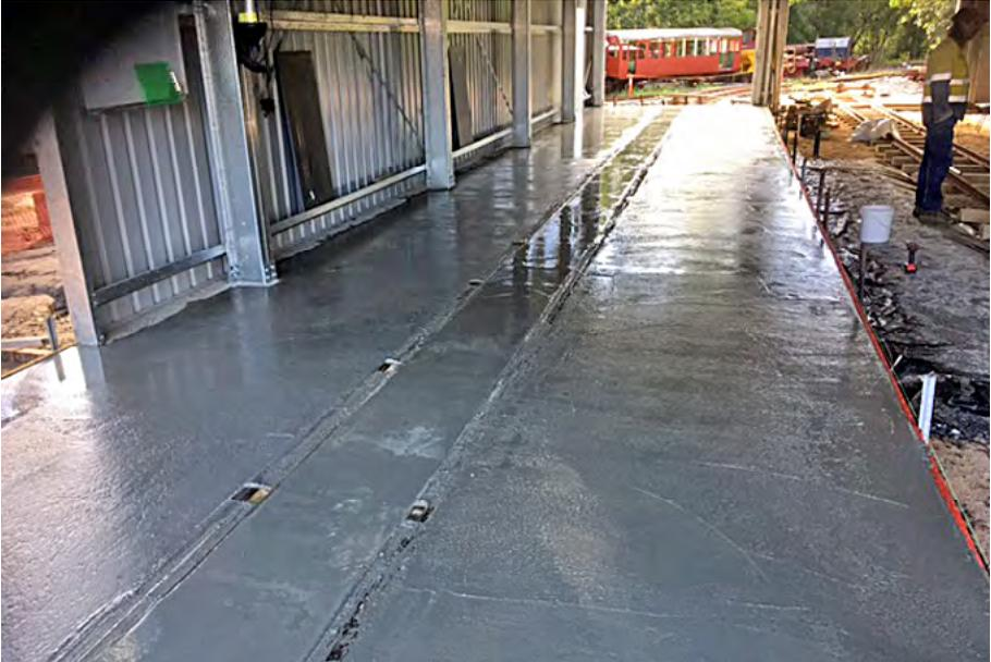
Greg Stephenson was on site to see the first section of concrete poured for the new loco shed floor, 3 April 2017. The outside track on the other side was poured the following day. The spacers for the flangeways were removed after the concrete hardened. Greg Stephenson photographer.
