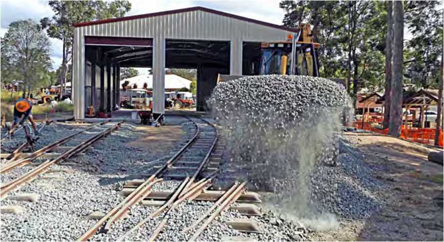
Ralph Cumner using his backhoe to transport and place ballast on Number 3 road. To reach this location, he travelled through the shed and along the track, 10 June 2017. Greg Stephenson photographer.
