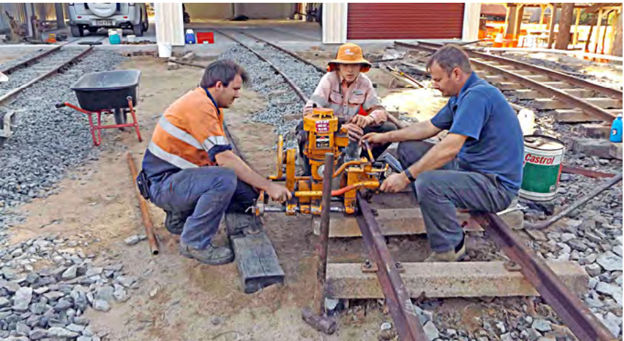
Ryan Thomas, Harrison Silk and Wayne Harman using the rail drill to make fishplated joints on Number 2 road, 3 June 2017. Greg Stephenson photographer.
