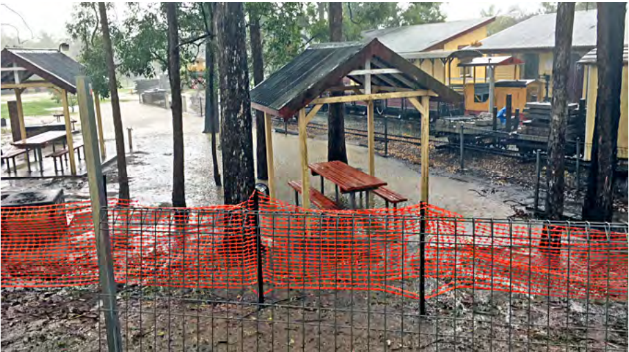
Picnic area from side door of locomotive storage shed showing rainwater flows, 14 October 2017. Greg Stephenson photographer.
