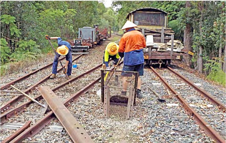
Sleeper renewals on the connection from the mainline to the workshop: Harrison Silk removes dog spikes while Terry Olsson and Dave Caruzzo remove ballast (and sift to remove dirt and small stones for reuse) from around the sleepers. In the foreground, the long steel sleeper to replace the point timber sits on the rail. Greg Stephenson photographer.
