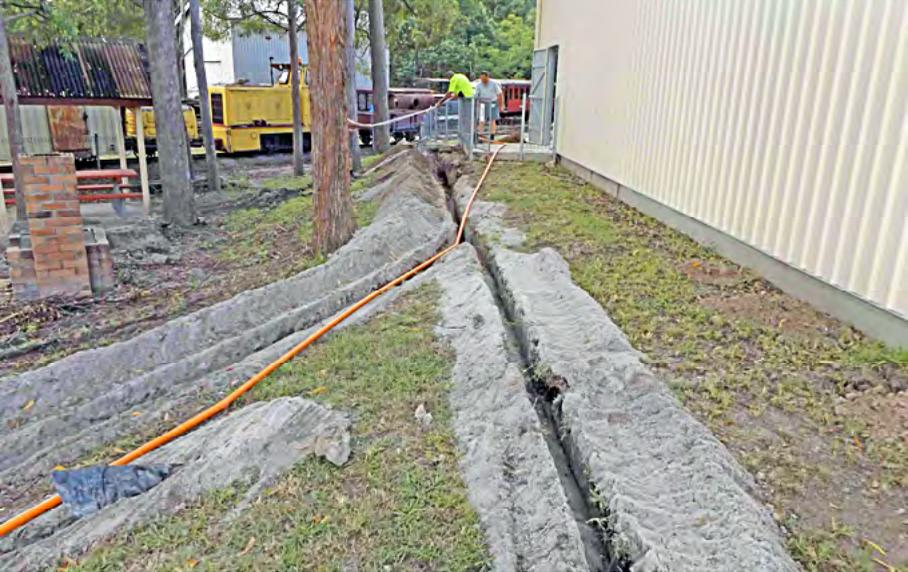
Drawing electric cables through orange conduits to provide power to the Locomotive Storage Shed, 20 March 2018. Greg Stephenson photographer.
