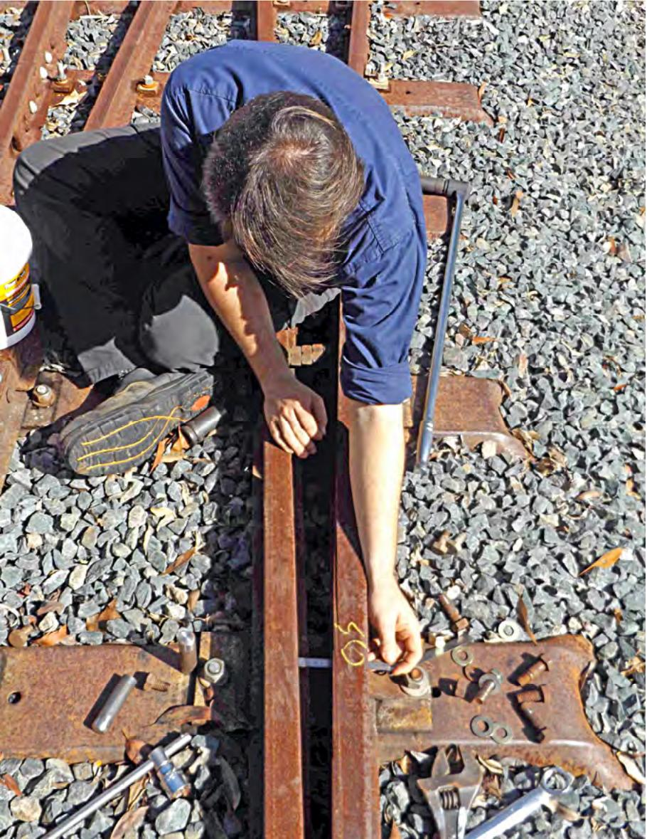
Ryan Thomas checks the length required before fitting the switch stops to the points leading to the Locomotive Storage Shed, 7 April 2018. Greg Stephenson photographer.
