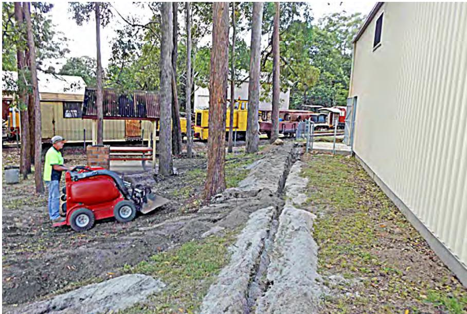
Once the cables and conduits had been placed into the trenches to provide power to the Locomotive Storage Shed, "Dingo Pete" returned to backfill the trenches, 20 March 2018. Greg Stephenson photographer.
