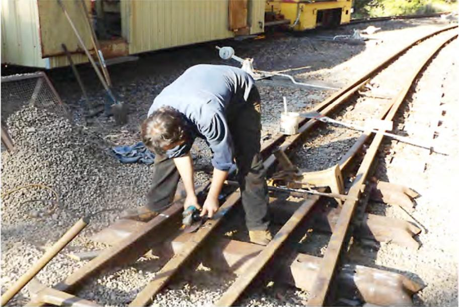
With 3 steel sleepers in place, Ryan Thomas prepares to install the shoulders for the Pandrol clips. A track jack has been inserted between the rails to hold them to gauge until the Pandrol clips are installed. Greg Stephenson photographer.
