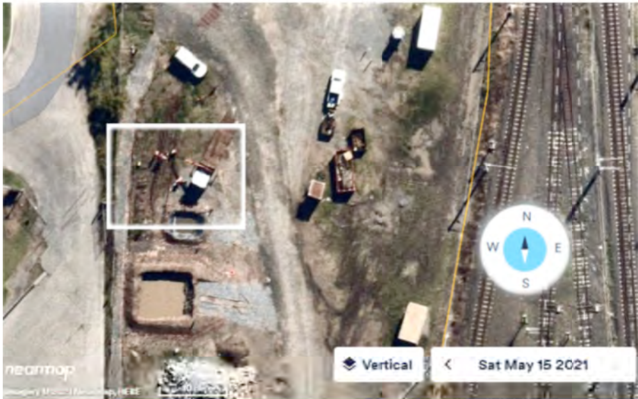
Nearmap imagery showing ANGRMS work party (outlined area above) removing the points at Clapham Yard, Yeerongpilly, 15 May 2021.
