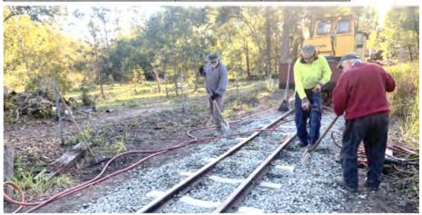
Packing, levelling and shaping ballast on an area of sleeper renewals at the start of Freeman's Cutting, Ryan Thomas photographer.
