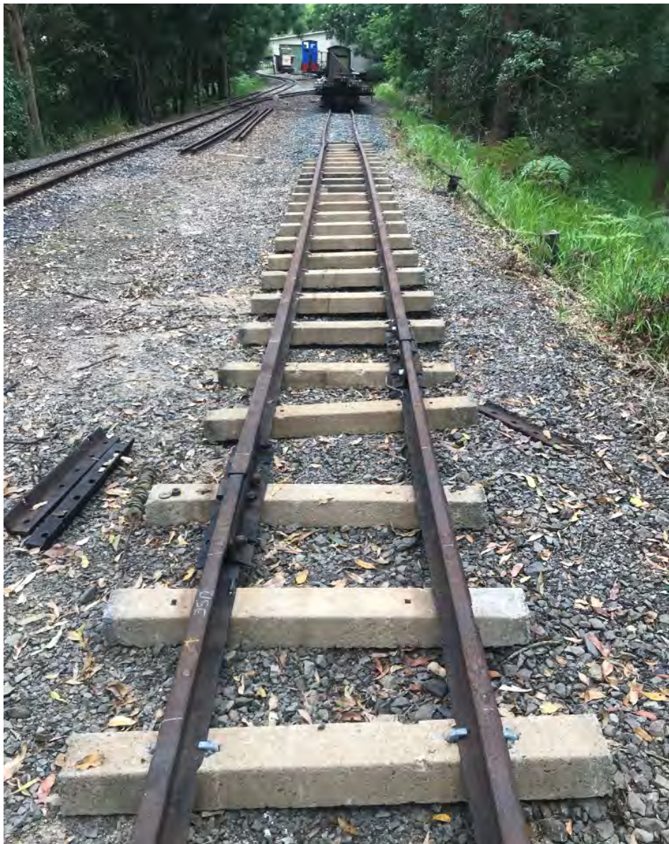
Re-sleeping and part re-railing the Workshop headshunt, 24 December 2022. Terry Olsson photographer.
