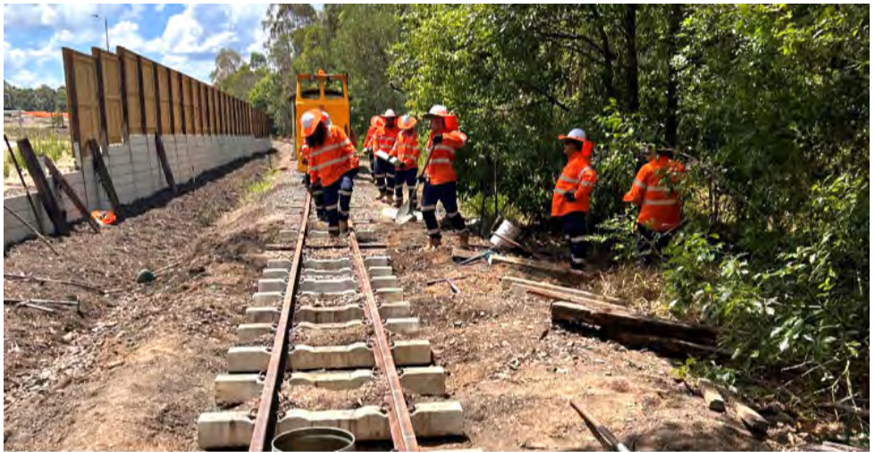
Track Course resleepering mainline near 550m mark. 5 December 2022. R Thomas photographer.
