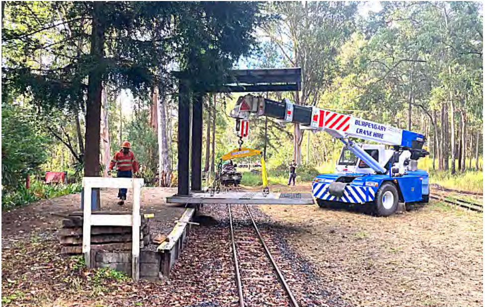
Placing first bus shelter module onto Peterson Road Station, 14 May 2024. Greg Stephenson photographer
